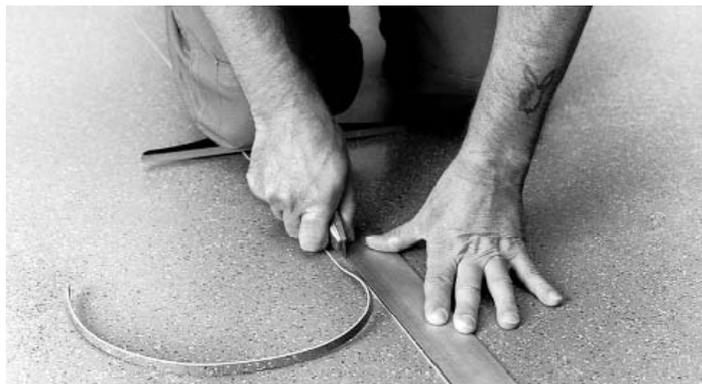
1. When double cutting the seam, use a straight edge as a guide. Position the straight edge about 1/2" (0.5") from the top edge. Cut through the top sheet and approximately 3/4 of the thickness of the bottom sheet using a utility knife and a sharp straight blade. When making the cut, hold the utility knife as vertical as possible
