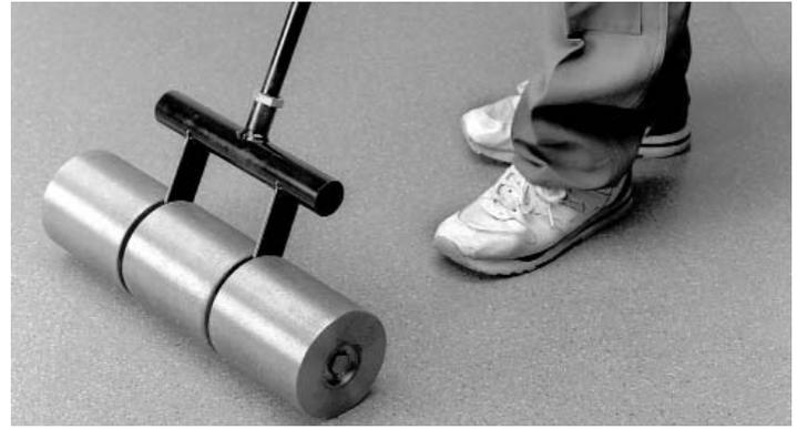
9. After one hour, re-roll the entire area in both directions with a 100 lb. roller
