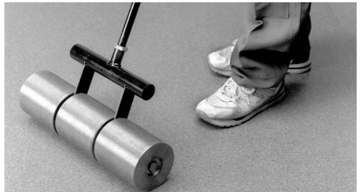
5. Roll slowly with a 100 lb. roller. Roll in both directions and avoid trapping air.
