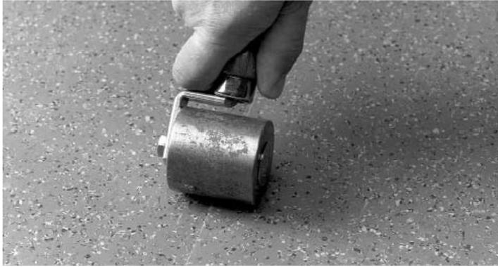
6. If required, hand roll seam area gently with a hand roller to smooth seam. Do not press hard with hand roller.
