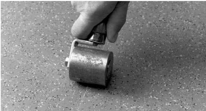
6. Only if required, hand-roll the seam area gently with a hand roller to smooth seam. Do not press hard with hand roller.
