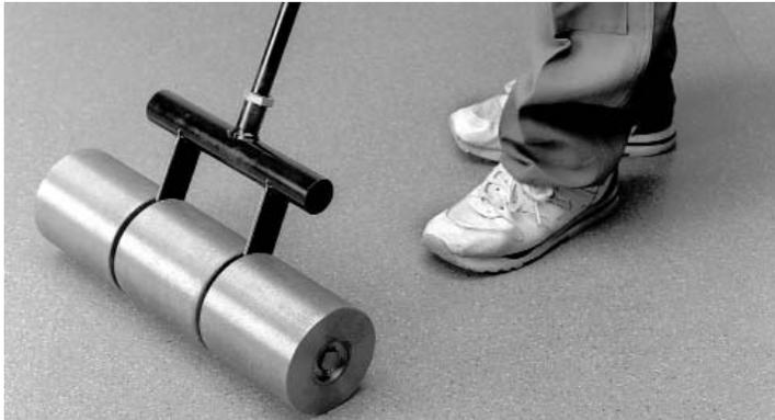
8. After one hour, re-roll the entire area in both directions with a 100 lb. roller.
